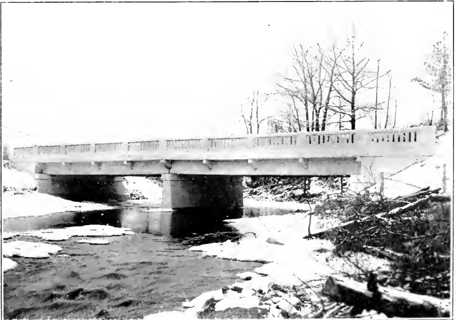
Black Creek Bridge, Highway No. 7, West of Actinolite.
